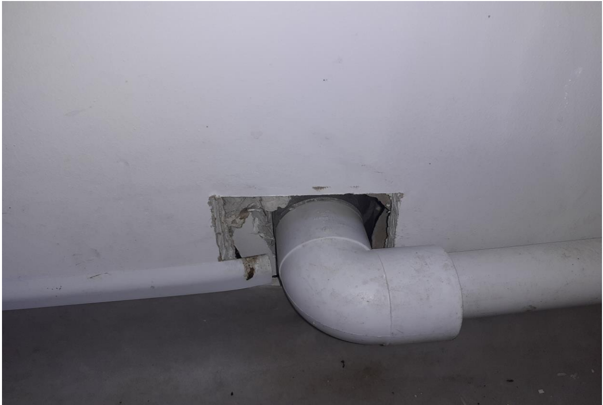
Gap round a pipe in the dry store room.
