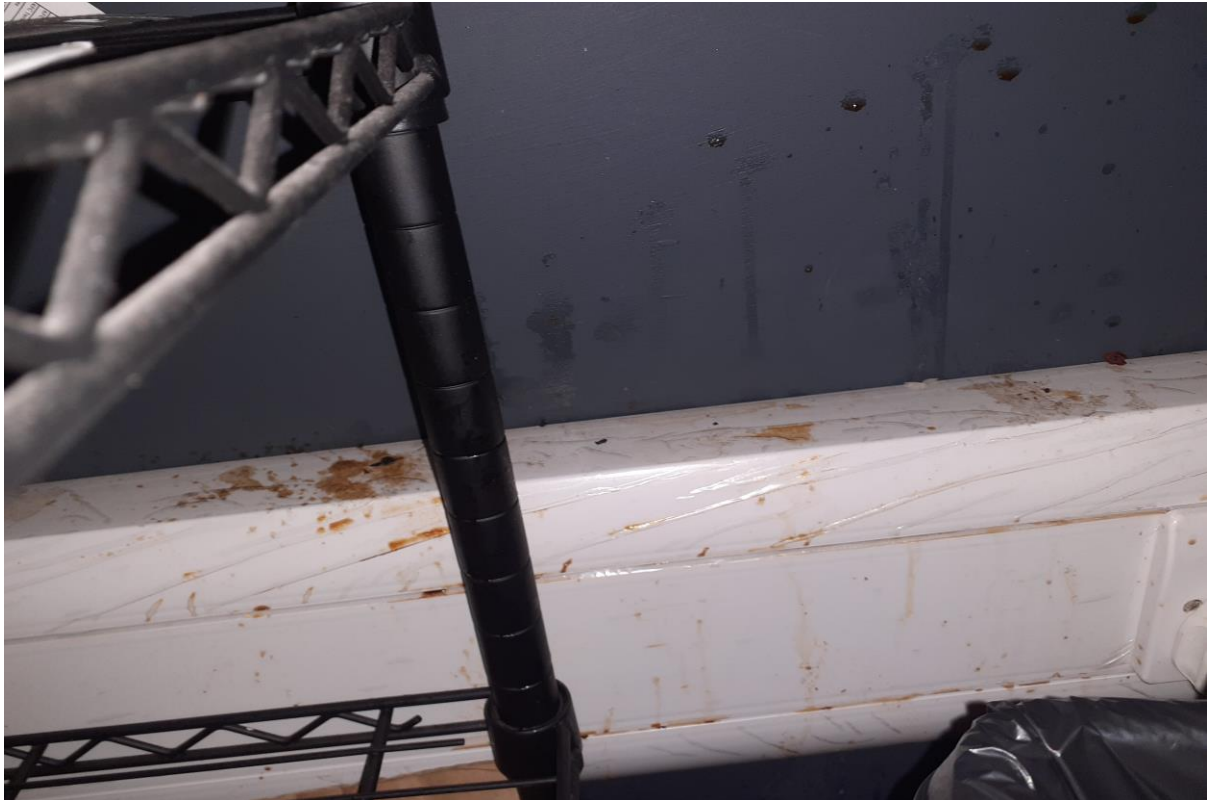
Dirty and mouse droppings on the electric trunking in the corridor area under the tills.
