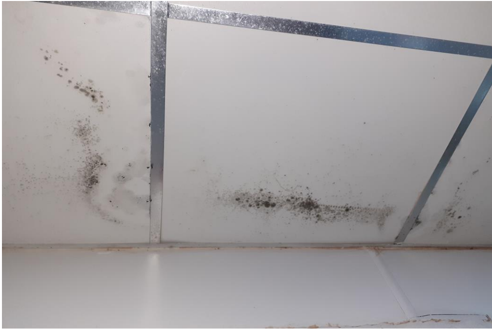
The ceiling was mouldy in front of the walk-in chiller in the rear preparation room.
