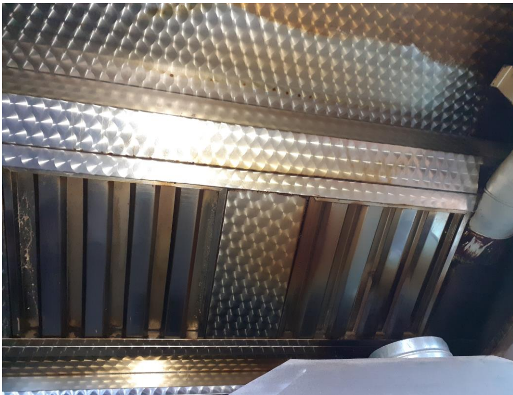
The filters in the ventilation canopy in the bakery area were dirty.
