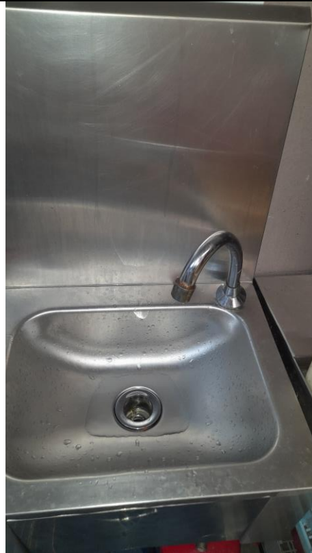
22. Wash basin next to pot wash area coming away from the wall
