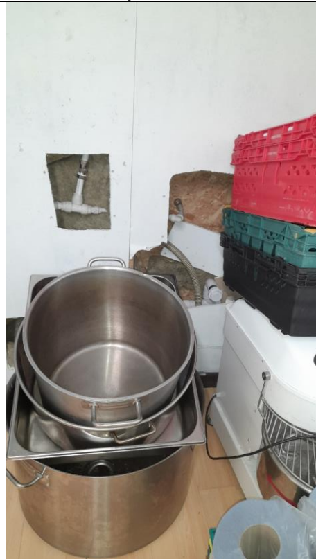
16. Holes to the wall behind the dough mixer and other equipment in the storage area
