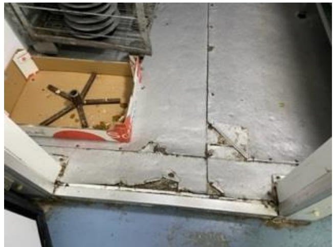
Photo 26 – Paint wearing off floor surface in first floor preparation area
