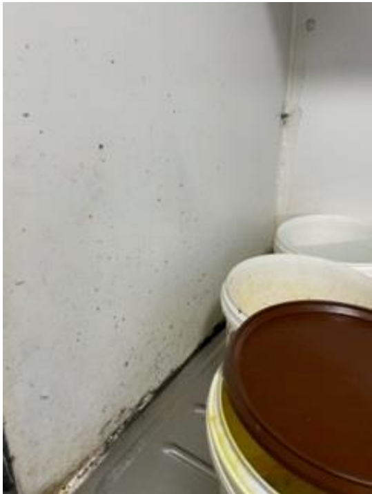
Photo 3 – Mouldy plastic partition wall surface to left of sink.
