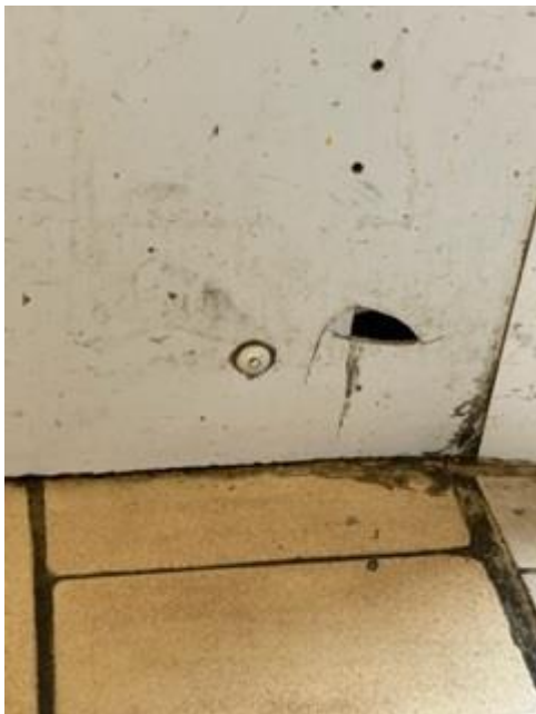
Photo 15 – Dirty damaged kitchen wall by sink area.
