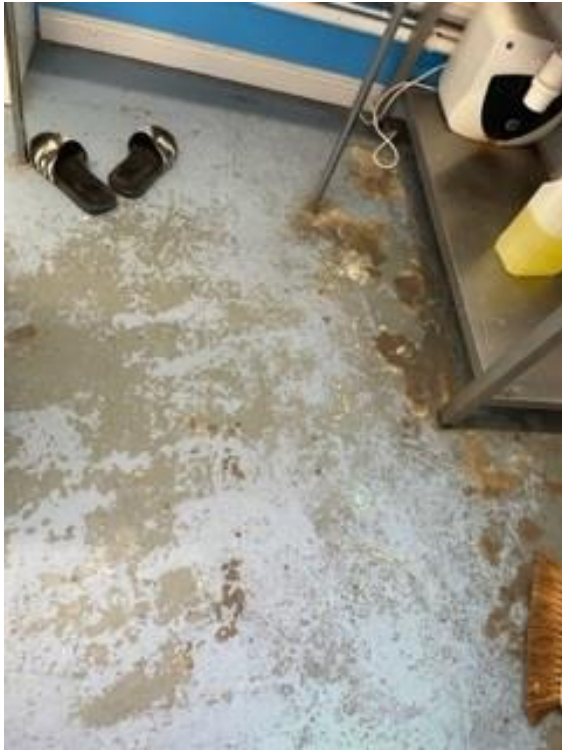
Photo 25 – Paint wearing off floor surface in first floor preparation area.
