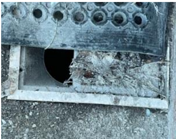
Photo 19 – missing external drain cover.
