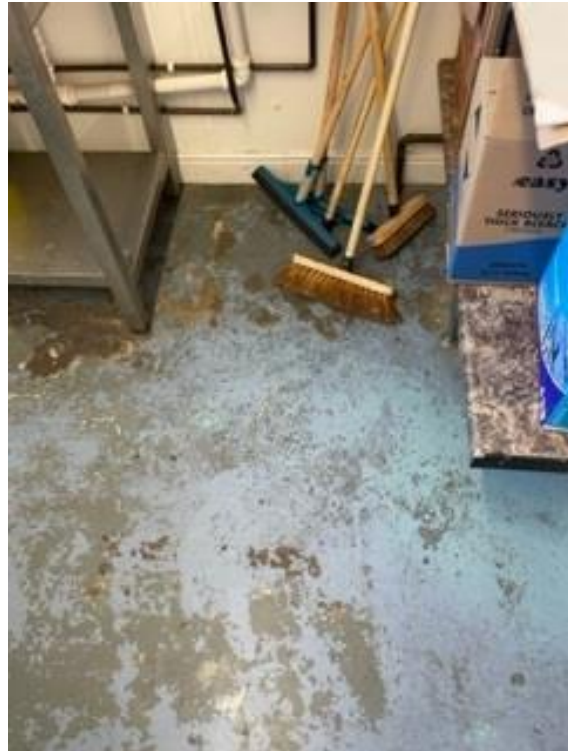
Photo 26 – Paint wearing off floor surface in first floor preparation area
