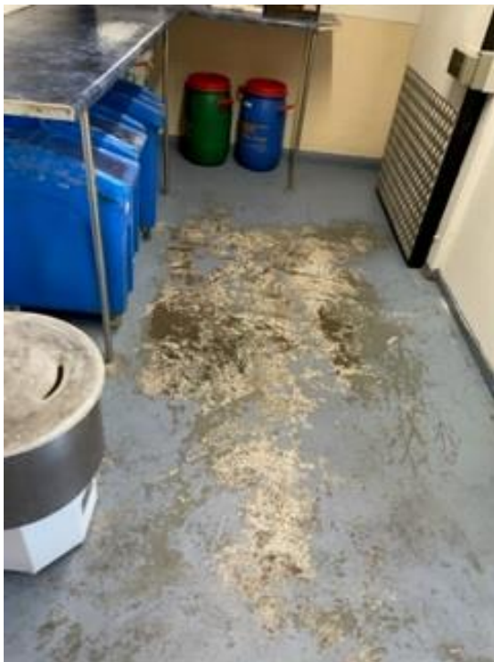
Photo 27 – Paint wearing off floor surface in first floor preparation area
