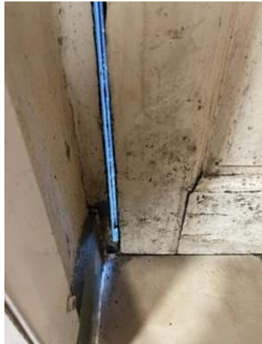
Photo 22 - Dirty rotten/ill fitting back door. When locked there are gaps which could allow mice into the business.
